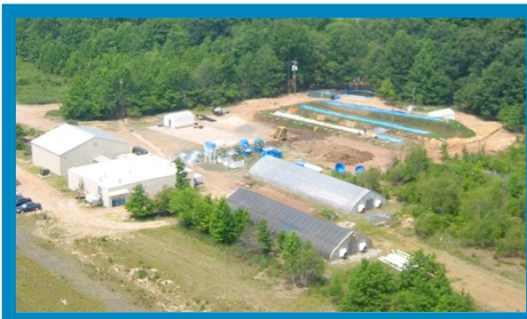
Urban Watershed Research Facility
