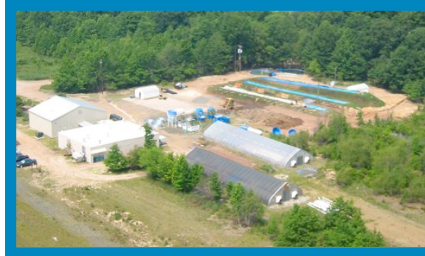
Urban Watershed Research Facility
